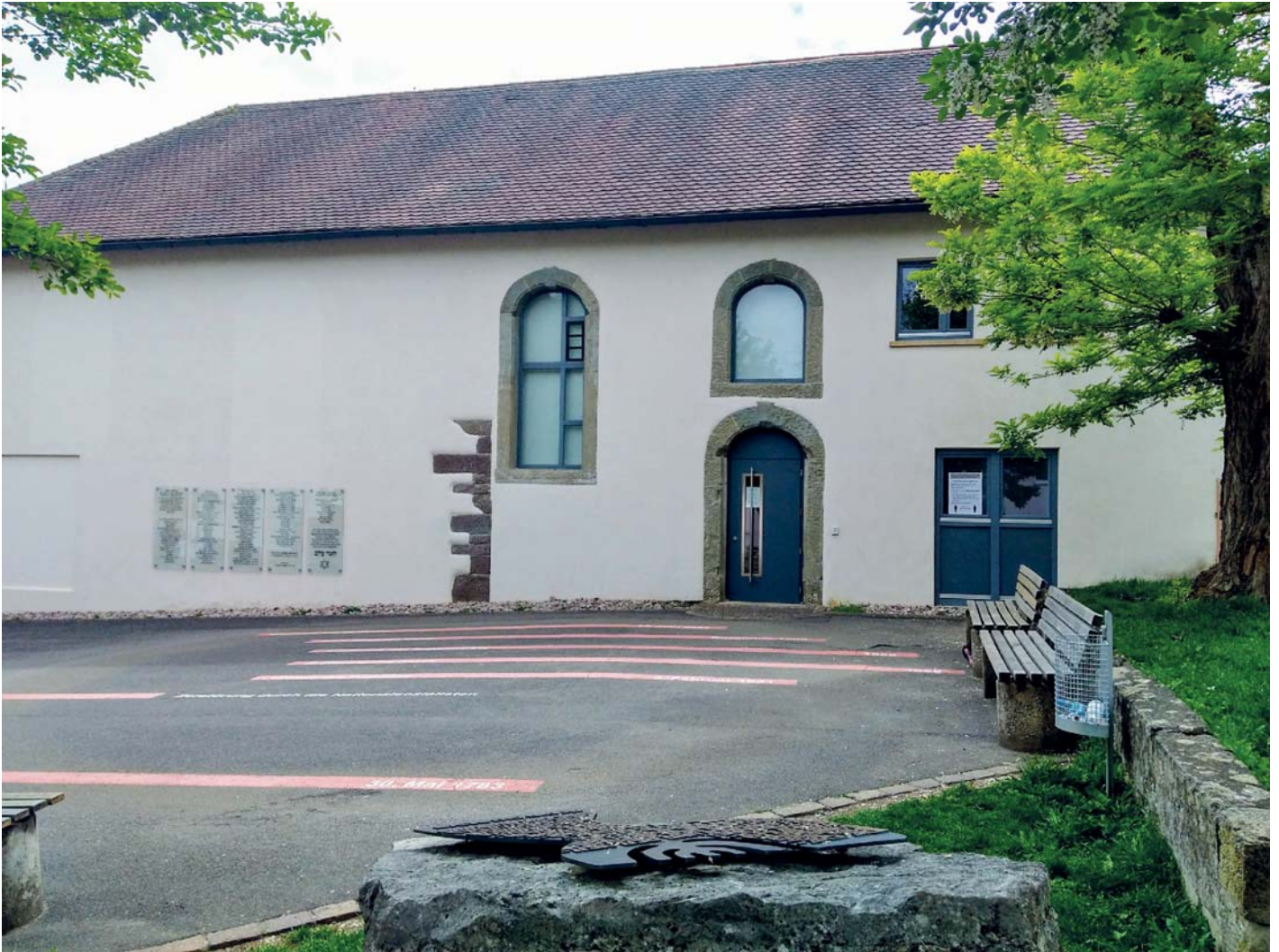
Outside view of the former synagogue. The commemorative stone with the seven-armed candelabra can be seen in the foreground on the right. The commemorative plaques with the names of all the deported Jews of Haigerloch are displayed on the wall of the synagogue on the left.
